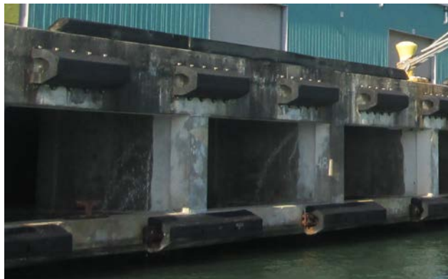
20"x6' Molded Arch and 20"x10' Extruded Trapezoid Fenders At Cargo Dock 14 & 15
