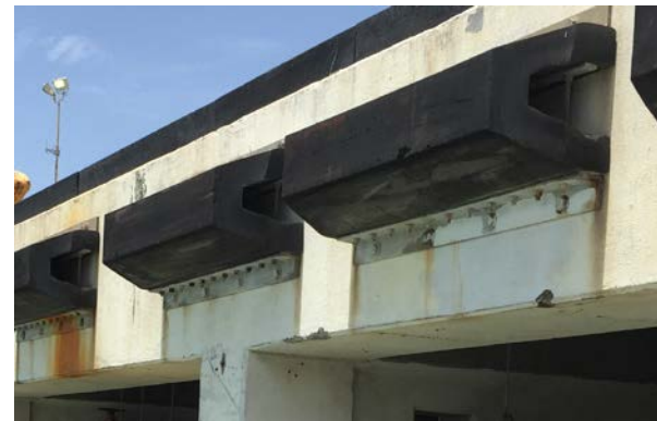
20"x6' Extruded Trapezoid Fender at Cargo Dock 9
